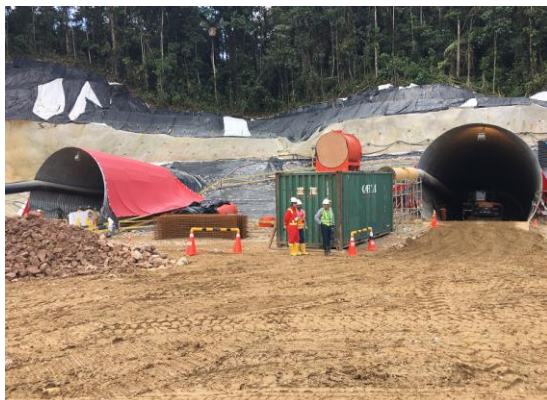
Lundin Gold: Twin Tunnels
